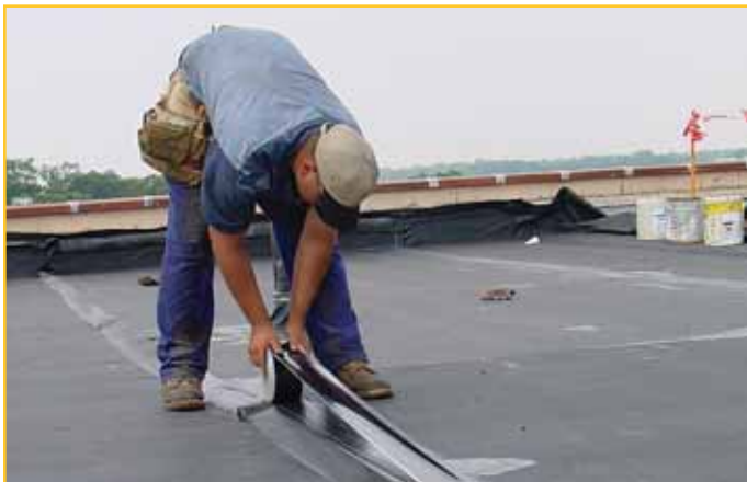
The old way of applying seam tape is time consuming and may cause injuries due to awkward positions.
