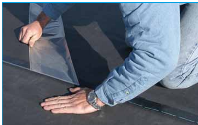
Seams completed with Versico's QAT Seam Technology go together smoothly, resulting in fewer wrinkles.
