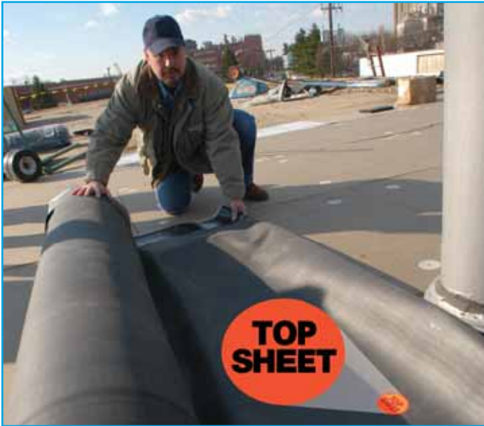
Locate the orange TOP SHEET sticker on 2-packs to ensure proper roll-out.
